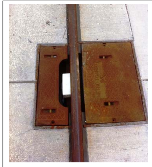
Fig. 5: Two examples of sensors protected from vehicular traffic. On the left is a wheel sensor at a steel mill protected from heavy trucks making nitrogen deliveries along the right-of-way. On the right is a sensor within embedded track on a light rail system.
