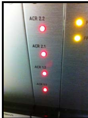
Fig. 23: AK19 Module assigned to two Binary Counter Modules with four channels in use. Red LEDs should illuminate when the ACR key is actuated.
